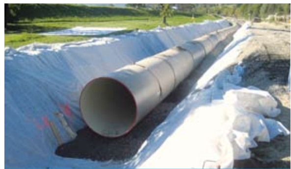
Laying of the discharge pipe
