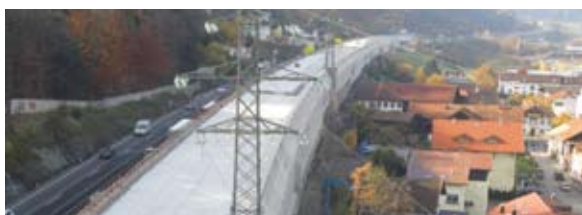
Electricity towers had to be raised because of the overhead noise barrier in the vicinity of Innsbruck/Amras
