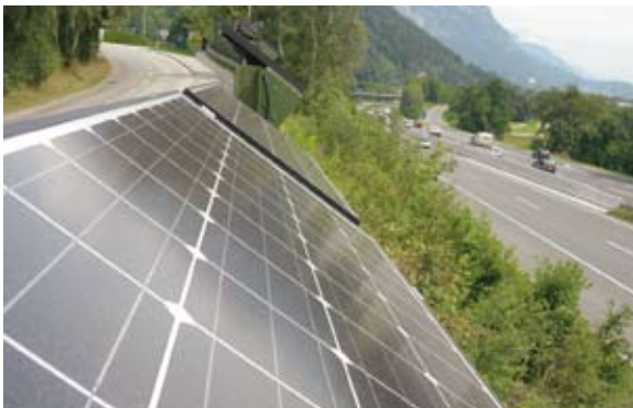
The photovoltaics station along the A12 in the vicinity of Vomp is mounted on the noise control barrier.
