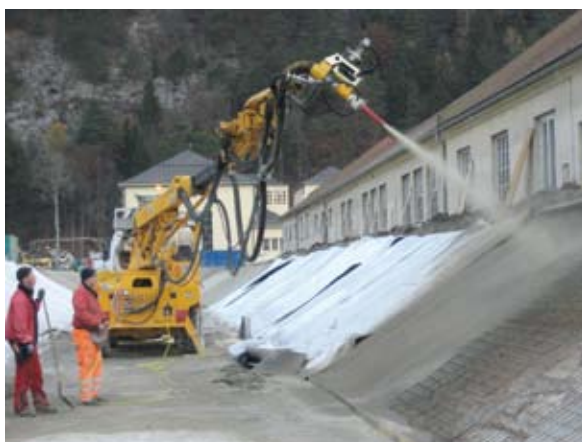
The embankments were renewed with the aid of a shotcrete robot.
